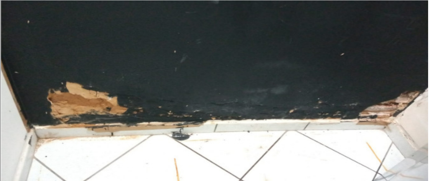
REBOCO DESAGREGANDO
