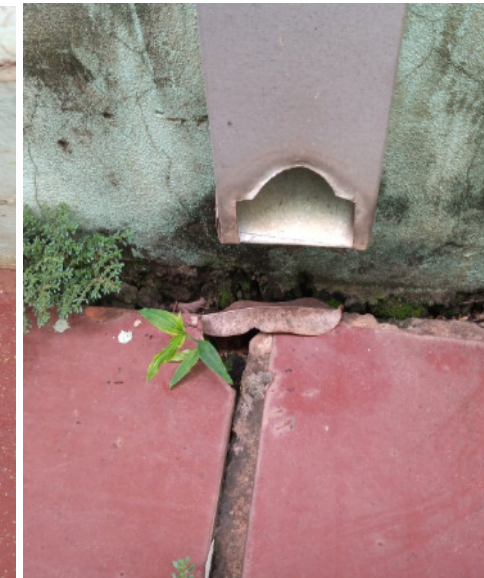
REBOCO DESAGREGANDO
