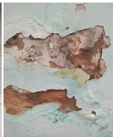
REBOCO DESAGREGANDO
